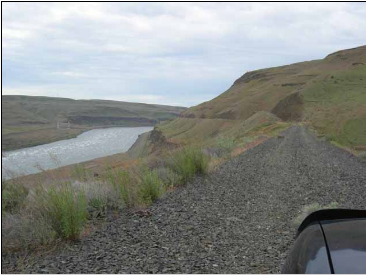
Figure 30. Large infills and bank cuts have disturbed and/or replaced native vegetation communities within the narrow WSPRC boundary along this portion of the trail.
