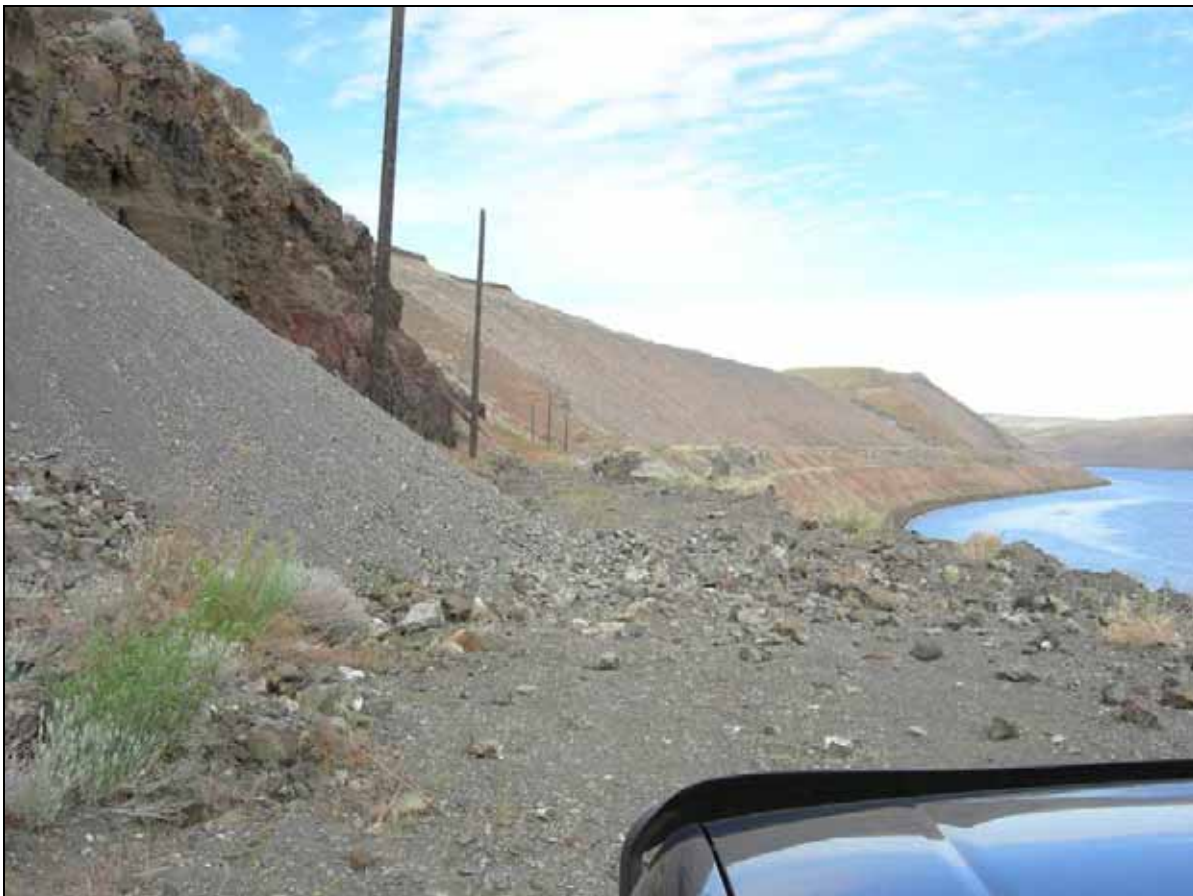
Figure 29. The CPT along this portion of the Snake River was dug out wide from the steep hillslopes above the river.
